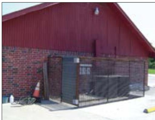
Example: This photograph illustrates AC units protected by a steel cage and security lighting.
